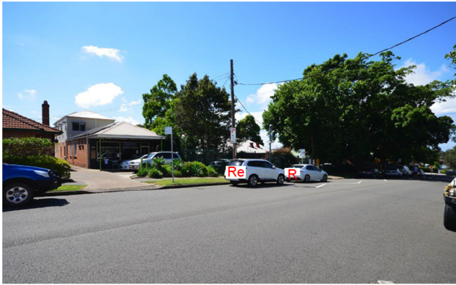
SMITH STREET - BUILDING OPPOSITE SITE (NORTH-EAST CORNER)
