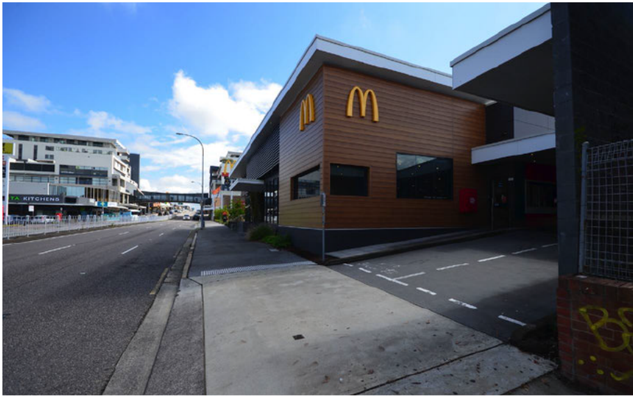
PACIFIC HWY LOOKING NORTH - NEIGHBOURING MCDONALDS BUILDING
