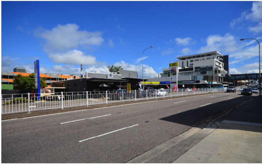
PACIFIC HWY LOOKING NORTH-WEST
